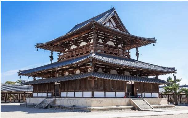
Figure 4 – The Golden Hall at the Hōryū-ji Temple. From ( Encyclopædia Britannica , by Andy M., n.d., Retrieved 2021, June, 9, from https://www.britannica.com/art/Japanese-architecture/images-videos#/media/1/719164/242133 ).
